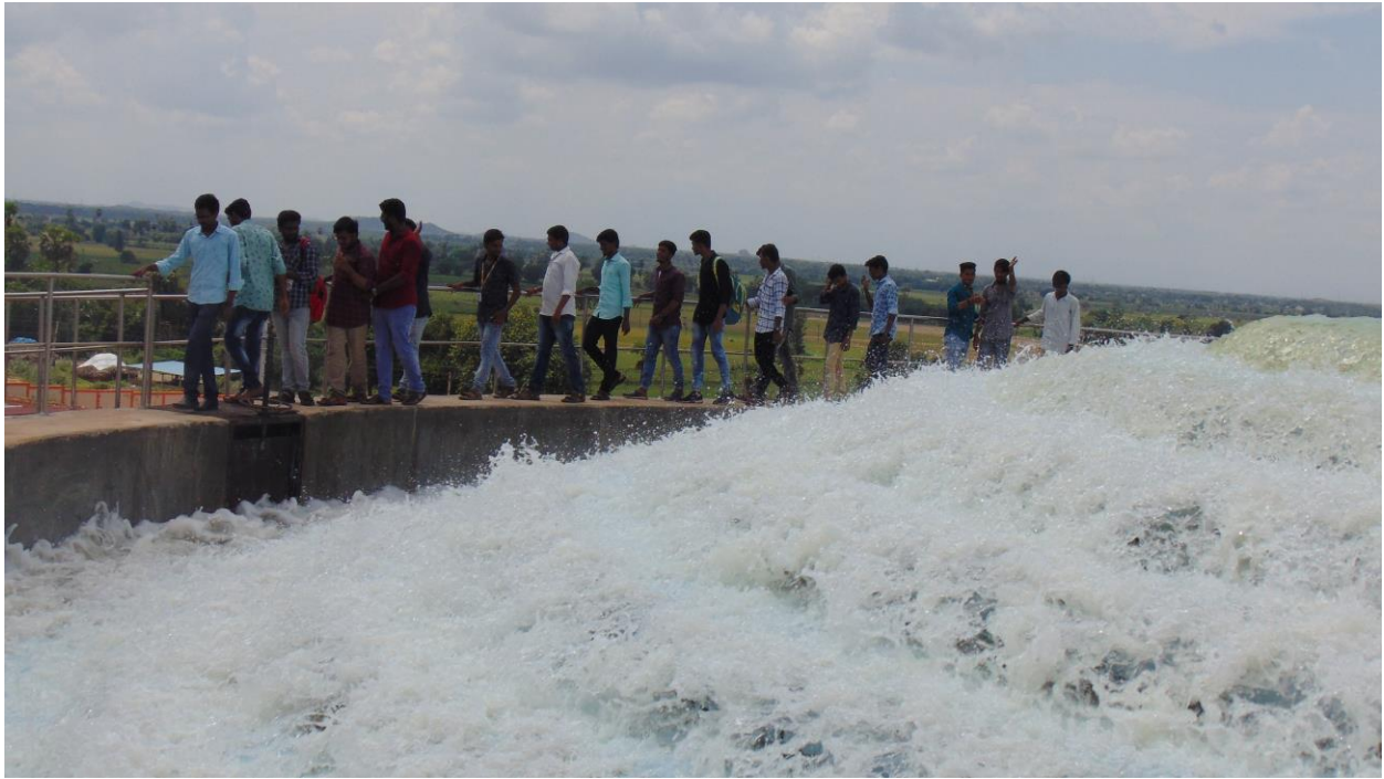
Students observing the Aeration tank
