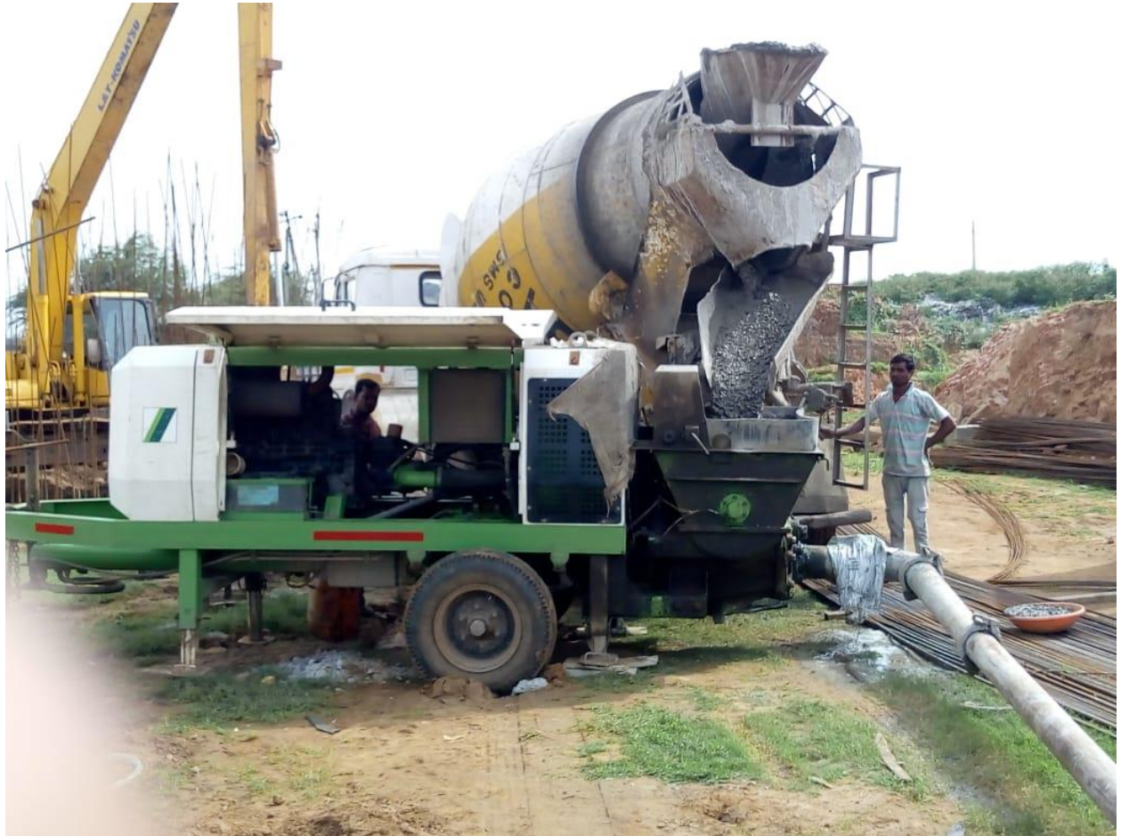
Loading Ready Mix
